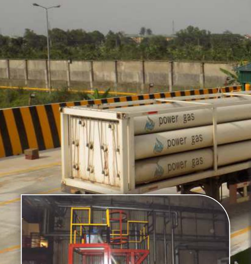
CNG plant installation 2
